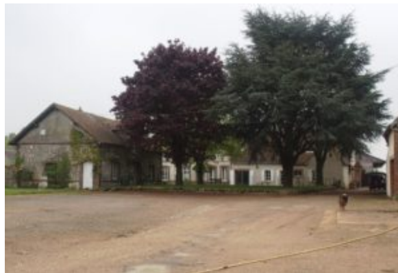
the dwelling house
